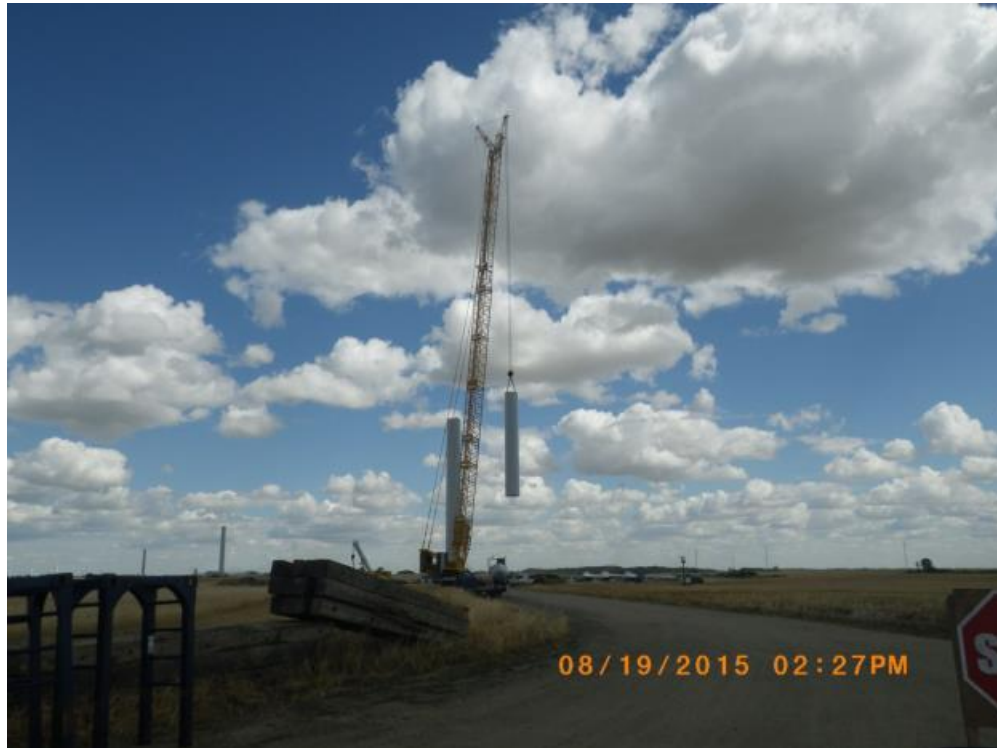
3. Tower Erection
